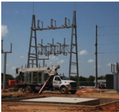
Construction during our Weldon substation project. The substation will be energized this month.
