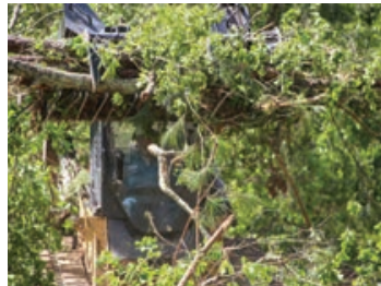
HCEC Crews use a skid steer with grapple attachment to easily pile debris.
