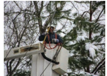
ROW Crews also utilize a bucket truck equipped with a hydraulic chain saw. The saws have a fiberglass pole to protect crews working near energized lines.
